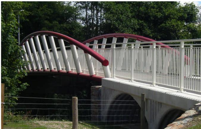
26 x 3m Vierendeel Bow String truss cycle bridge at Tavistock—Client Devon CC—Ref 3070
